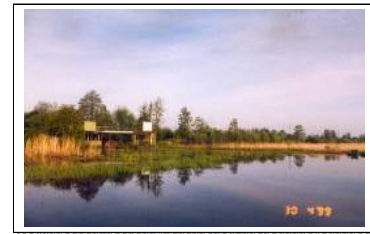
Station de pompage
